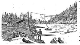
Typically in the early 1800's, river crossing ferries consisted of two docks connected by an overhead rope line to hold the raft crossing during the strong spring currents.
